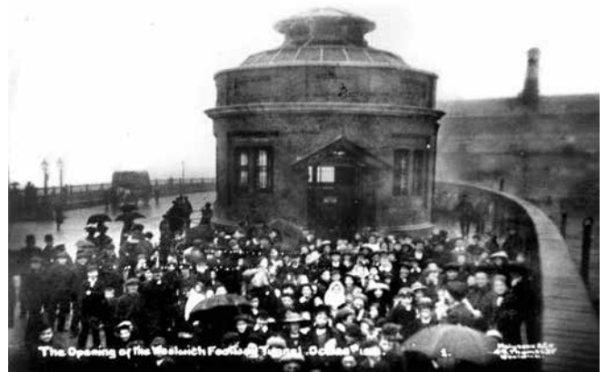
Despite heavy rain, crowds gather for the opening of the Woolwich foot tunnel on 26 October 1912
